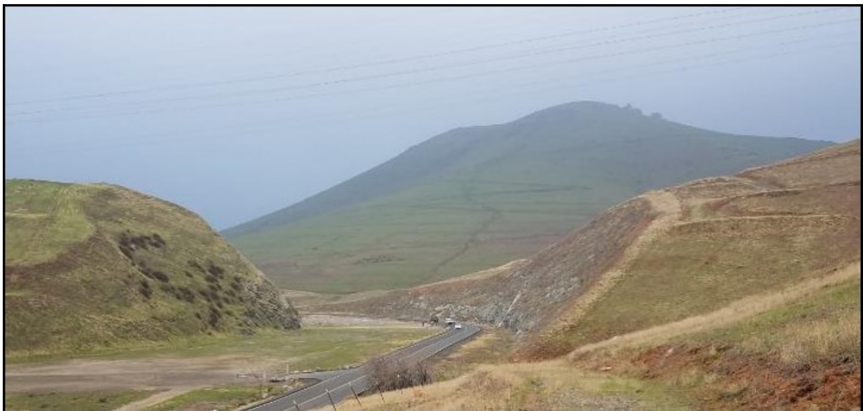
Figure 6. View of spillway from Lake Success. Phase 1 involves blasting and excavating the right abutment of the spillway. Worth Drive/Avenue 146 is adjacent to the right abutment.
