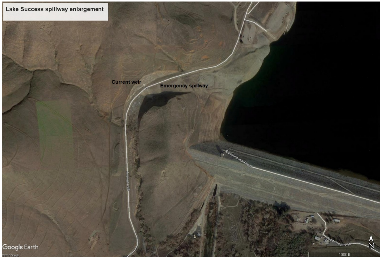
Figure 5. Overview of the emergency spillway on the southwest corner of Lake Success. The spillway will be widened 165 feet by blasting and excavating the right abutment (top side of the spillway in this figure). Worth Drive/Avenue 146 (white line) currently goes through the spillway and will be relocated onto a bench above the new, wider spillway.
